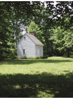
One of the buildings at historic Buck Spring; citizens are working to establish a regional conference center there.
